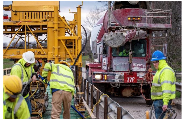
A construction crew pours a concrete deck for a bridge in Nelson County.
